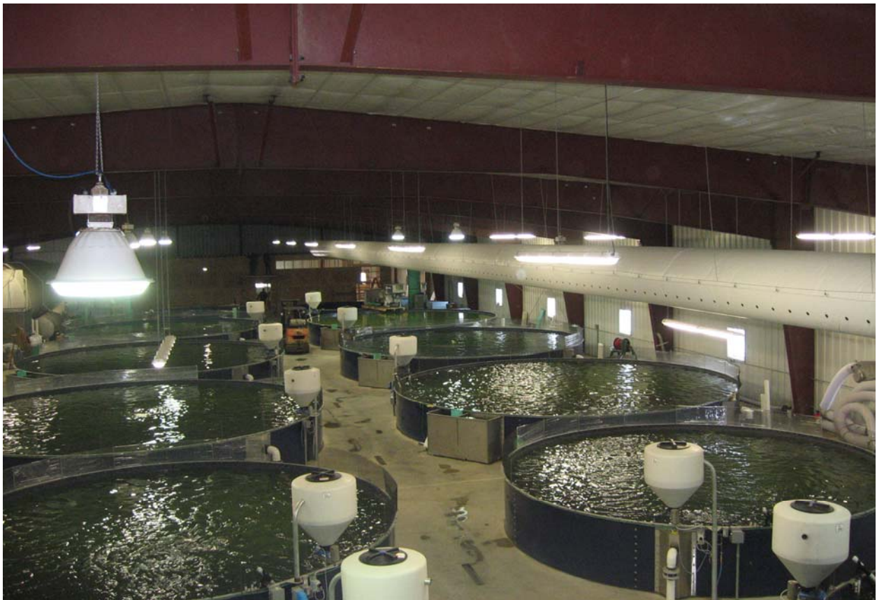
New Hutterite 300k lbs. Production Facility - Montana
